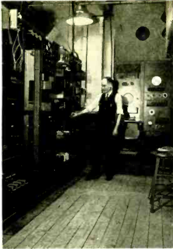
Television control room.
